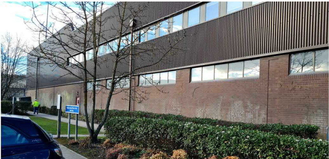
Plate 7.2 - Example of an Existing Building
