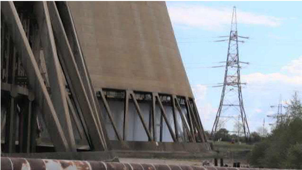
Plate 5.11 - Example of the Cooling Water Reservoirs
